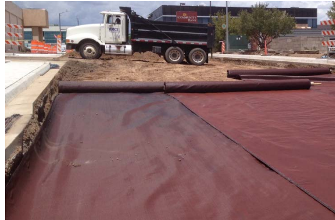
Image 7–Extending the Geosynthetic Reinforcement up a Vertical Face
