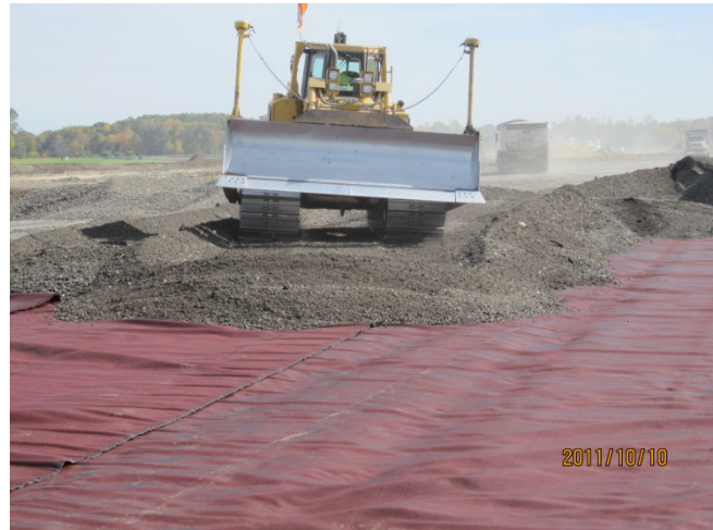
Image 4 – Spreading aggregate over geosynthetic
