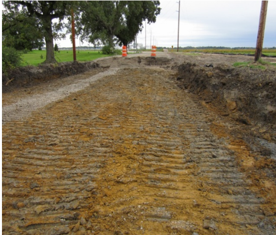
Image 1 – Subgrade Preparation
