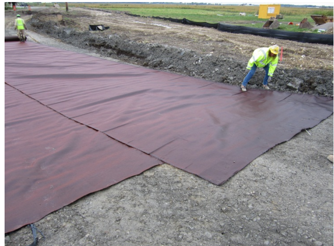
Image 2 – Geosynthetic Deployment
